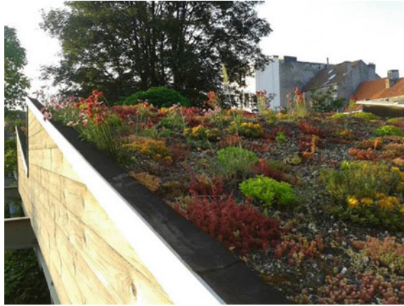
Fig. 6.8 Extensive sloped green roof (Berghem, Belgium)
