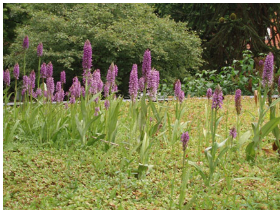
Fig. 6.7 Extensive flat roof planted with sedum. After 5 years the first establishment of native Orchids ( Orchis praetermissa ) occurred (photo H. van Bohemen, The Netherlands)
